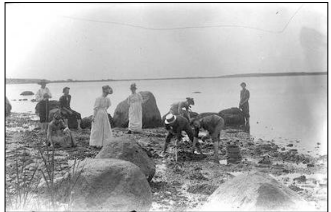
Digging for Clams in 1890's
